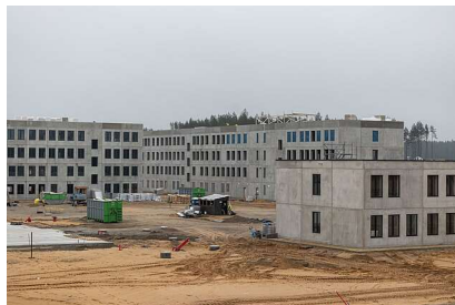
Construction work at the Rūdninkai military training area is progressing significantly faster than planned.
